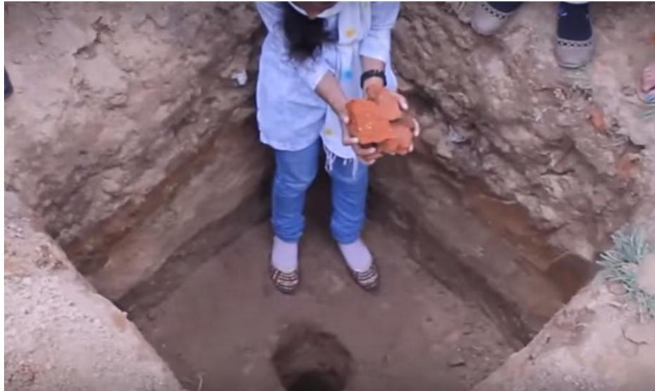
**Figure 13: Recharge pit & Soak pit preparation.**
