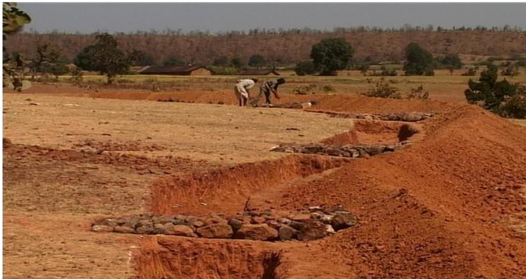
**Figure 10: Earthen contour bund.**
